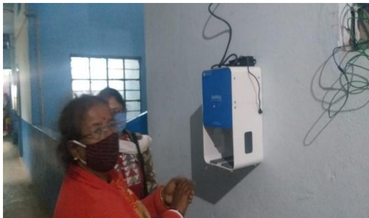
Installation of sanitizer dispenser machine (capacity 1.5L, Oakmist).
